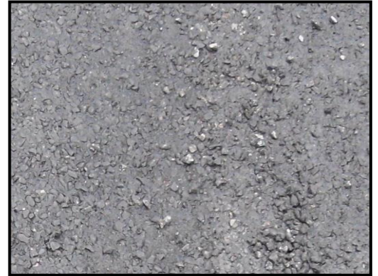
Surface Finish 1 day After Treatment
