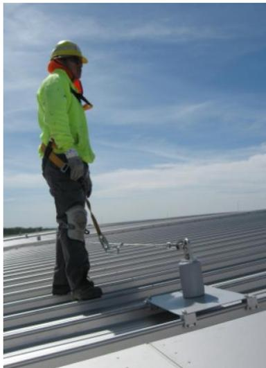
High Access Solutions Ltd have been contracted to install a Mansafe access system on the roof of the Blaise in-vessel composting facility. The system allows suitably trained employees to safely work on the roof areas at the facility while ensuring they are appropriately harnessed and anchored to secure points. Mansafe offers a number of benefits, including enabling routine and emergency maintenance of the air extraction system to be undertaken expediently.
